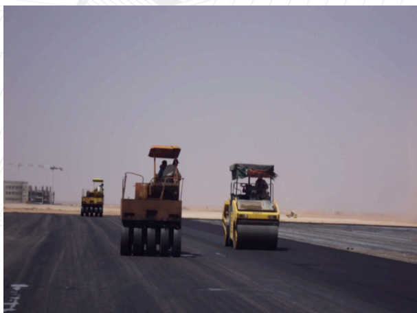
Asphalting of inner and local roads.
