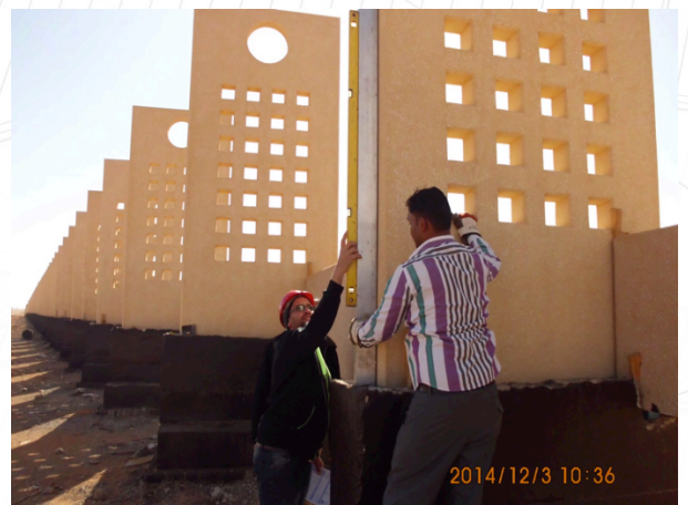
Erecting of pre-cast Panel for perimeter fence.
