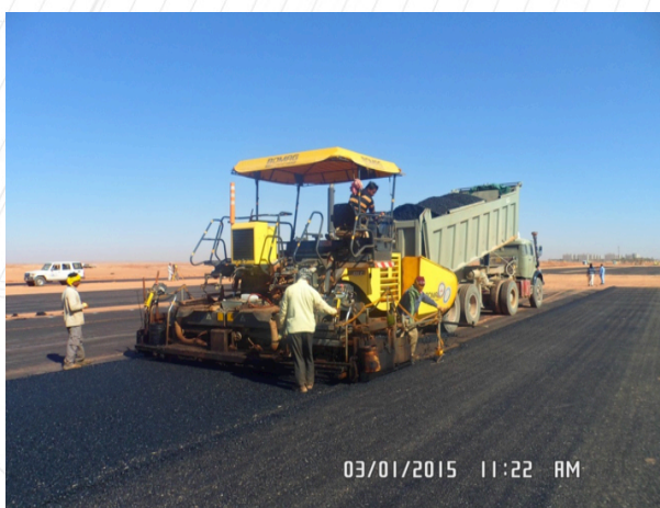
Asphalting of inside parking.
