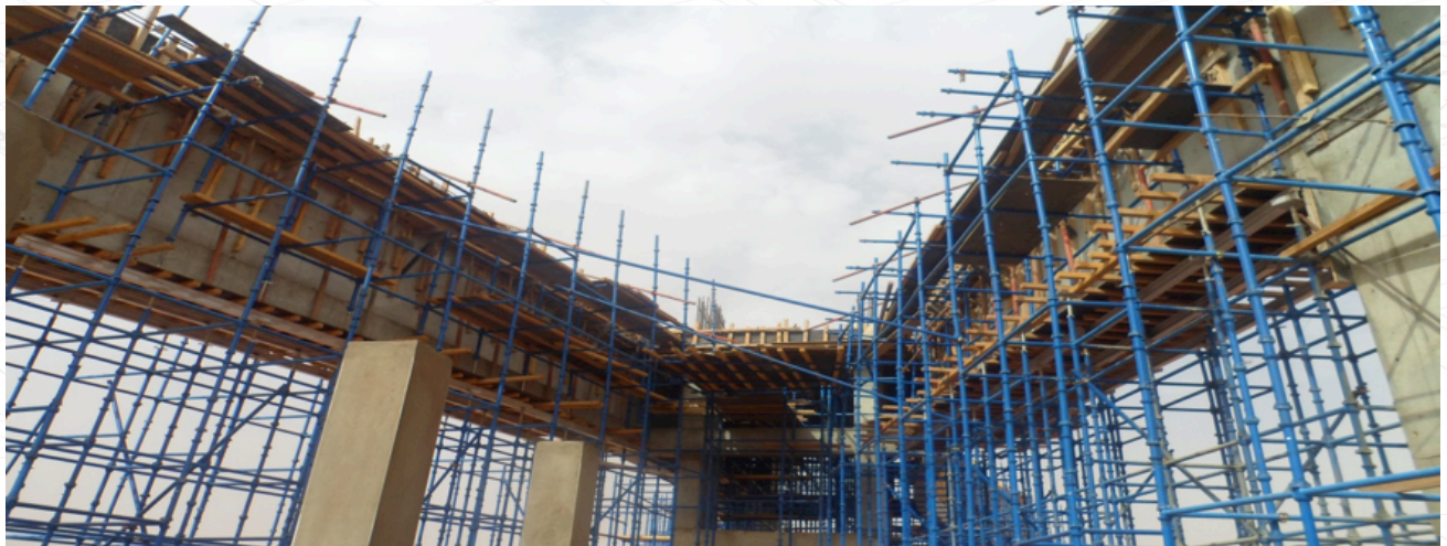
Formwork of Main Gate (2) of the University
